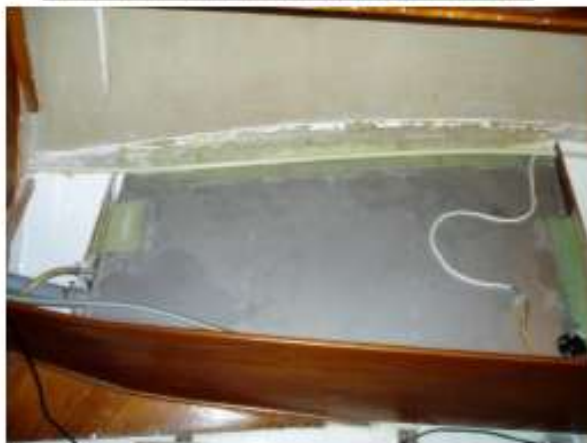
Cabin SB – New water tank mounted
